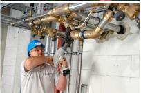
Viega's press technology saved additional time when installing the drinking water system particularly when laying the 8-km stainless steel pipe system Sanpress for the main distribution in the Allianz Arena. Since the XL dimensions between 76.1 and 108.0 mm could be reliably pressed in just a few seconds, vital seconds were saved before the whistle was blown for the opening match.
