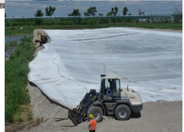
Remediation (Sludge Lagoon)
