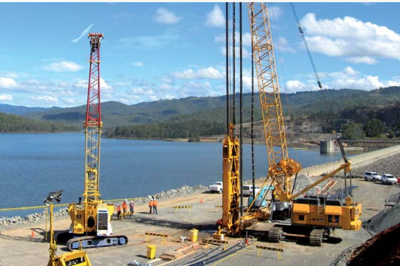
50 metre deep cut-off wall at the Hinze Dam in Australia
