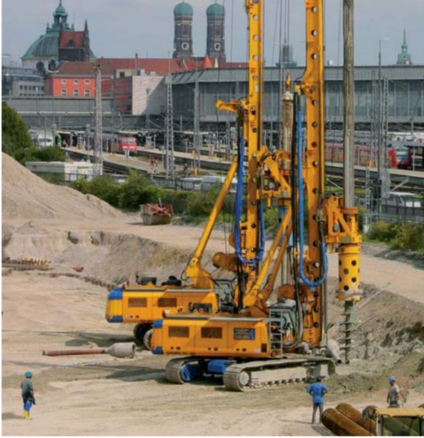
Retaining structure/foundations, Munich Central Bus Station
