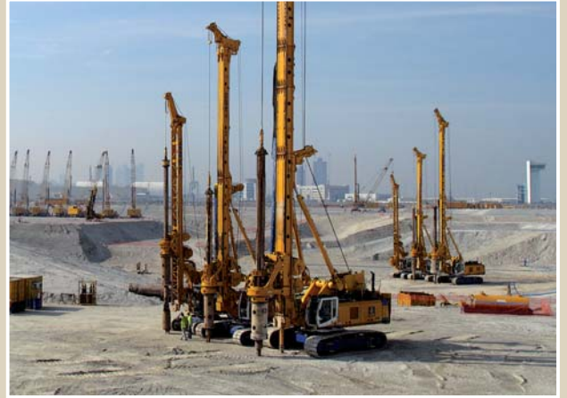
Excavation pit and foundations for the Louvre in Abu Dhabi
