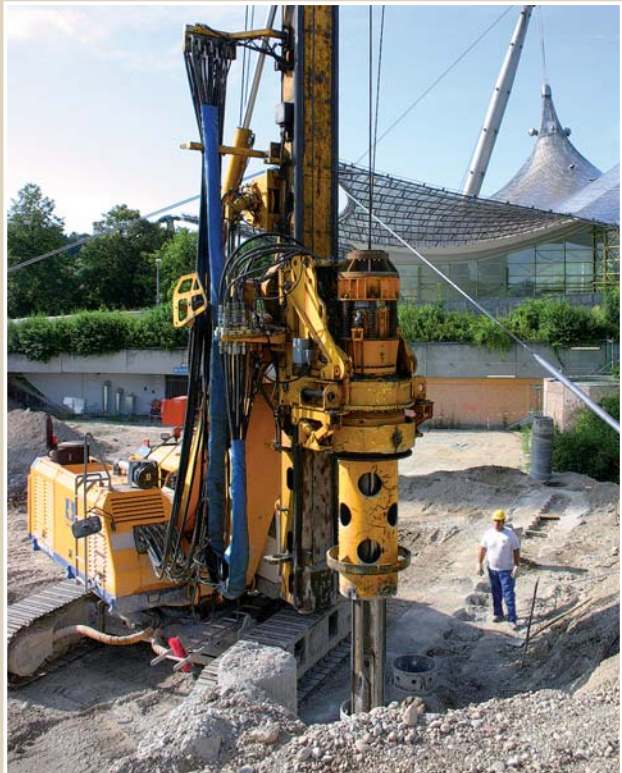
Reconstruction of the small Olympic Hall in Munich
