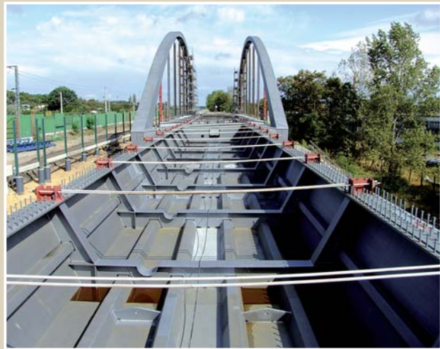
Schachtbau Nordhausen: Steel bridge over the Havel
