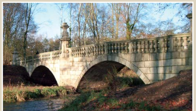
Muttone bridge in Waldsassen – renovated by Spesa
