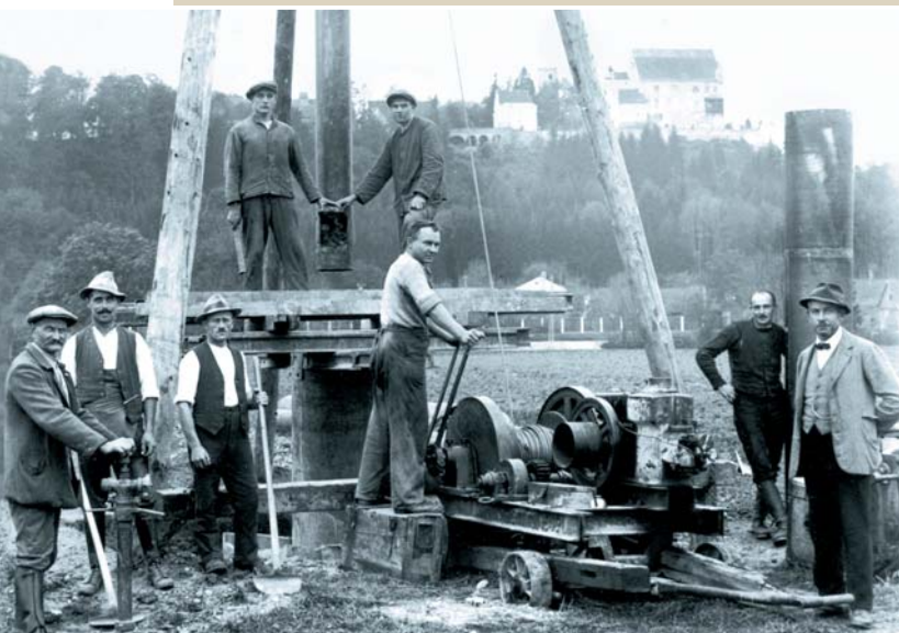
Well drilling using the tripod derrick, into the 1950s
