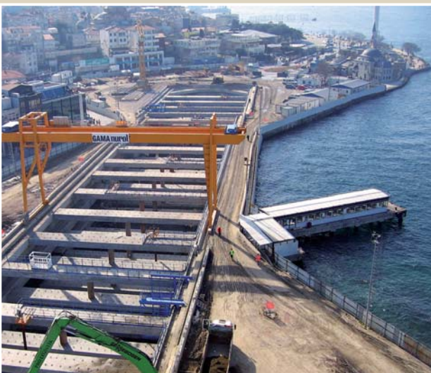
Excavation pit for metro line under the Bosphorus in Istanbul
