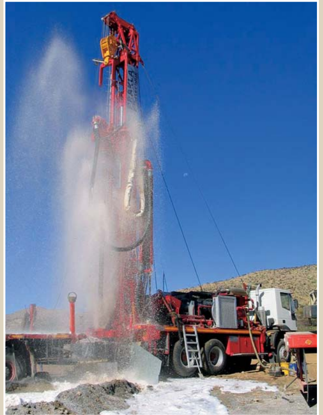
The Prakla RB 50 in operation – water supply in Namibia
