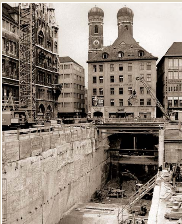
Marienhof excavation pit for the underground/overground rail crossing, Munich 1967
