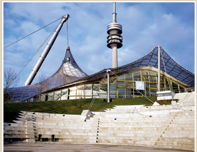
Bauer anchoring for the Munich Olympic Stadium's tent-style roof, 1972
