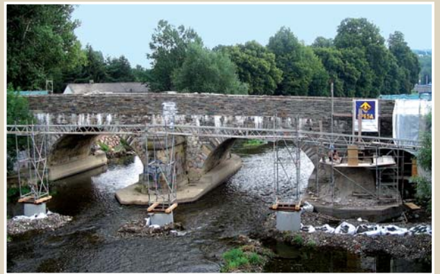
Renovation of the Alte Elster bridge in Plauen by Spesa
