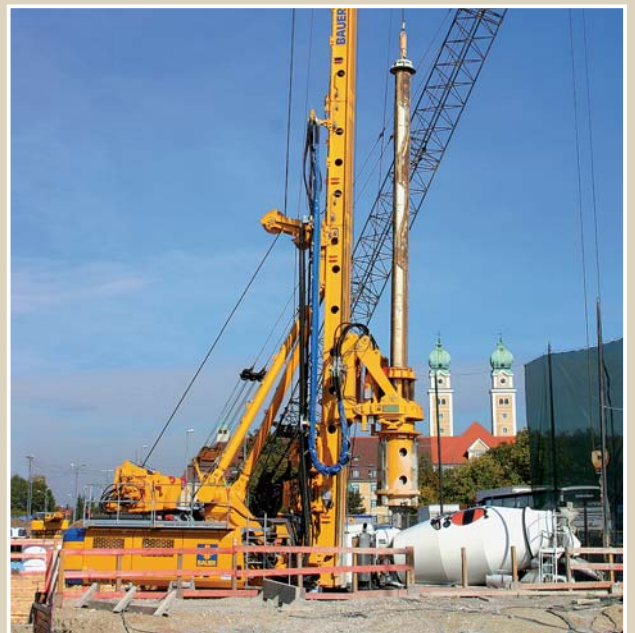
Tunnelling beneath Munich's Central Ring Road at Luise-Kiesselbach-Platz
