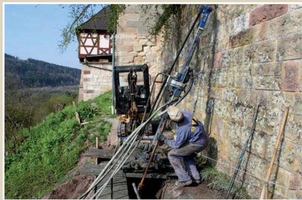
Masonry renovation by Spesa at the Lorch monastery
