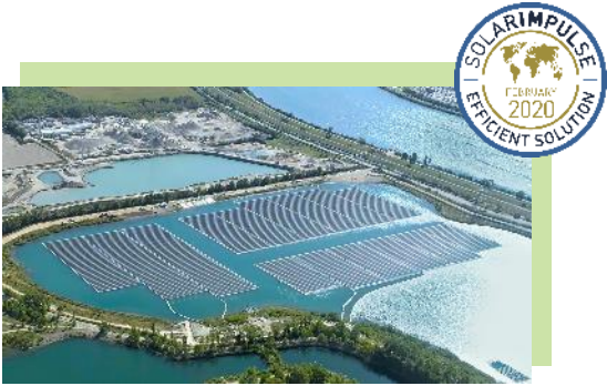
Floating solar (Hydrelio® by Ciel&Terre)
